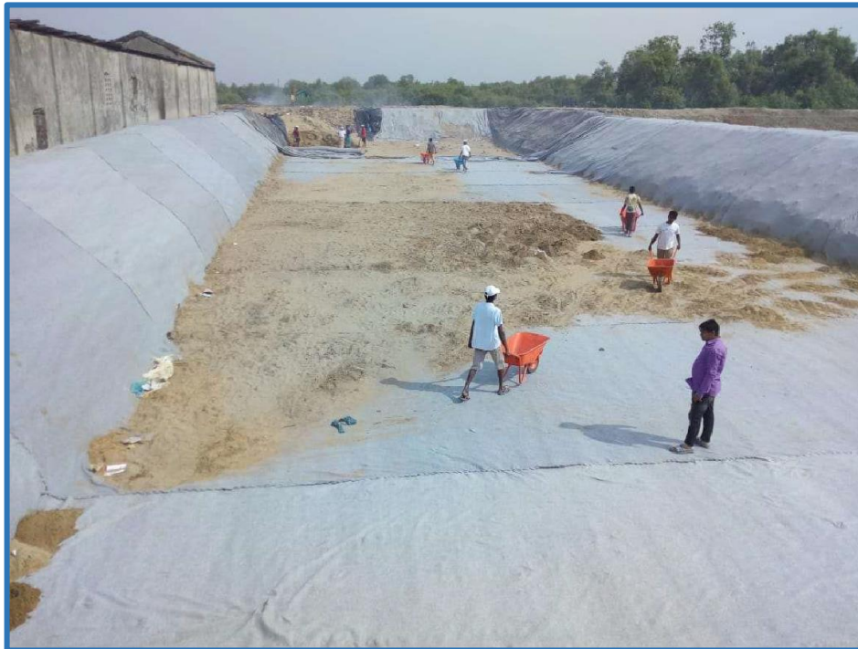
Figure 4 Temporary Solid Waste Facility at Ward 7, Teknaf Municipality
