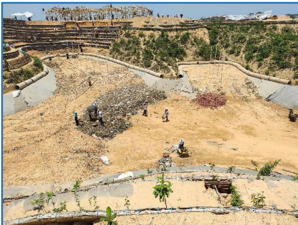
Figure 5 Temporary Solid Waste Facility (Landfill) at Camp20ext
